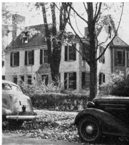
The Iktinos chapter house after the fire. The burned third floor is partly concealed by the trees.
