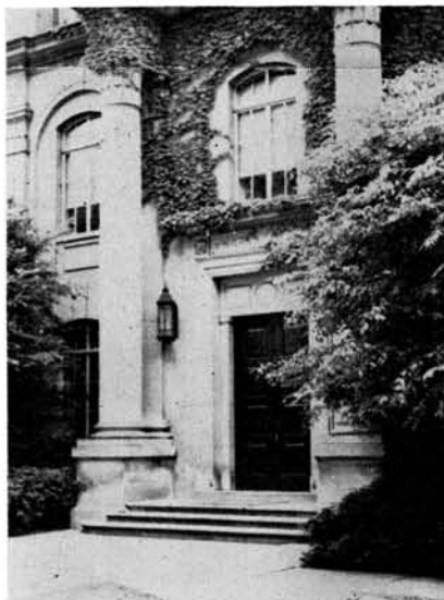
Engineering Building, The Pennsylvania State University, State College.
